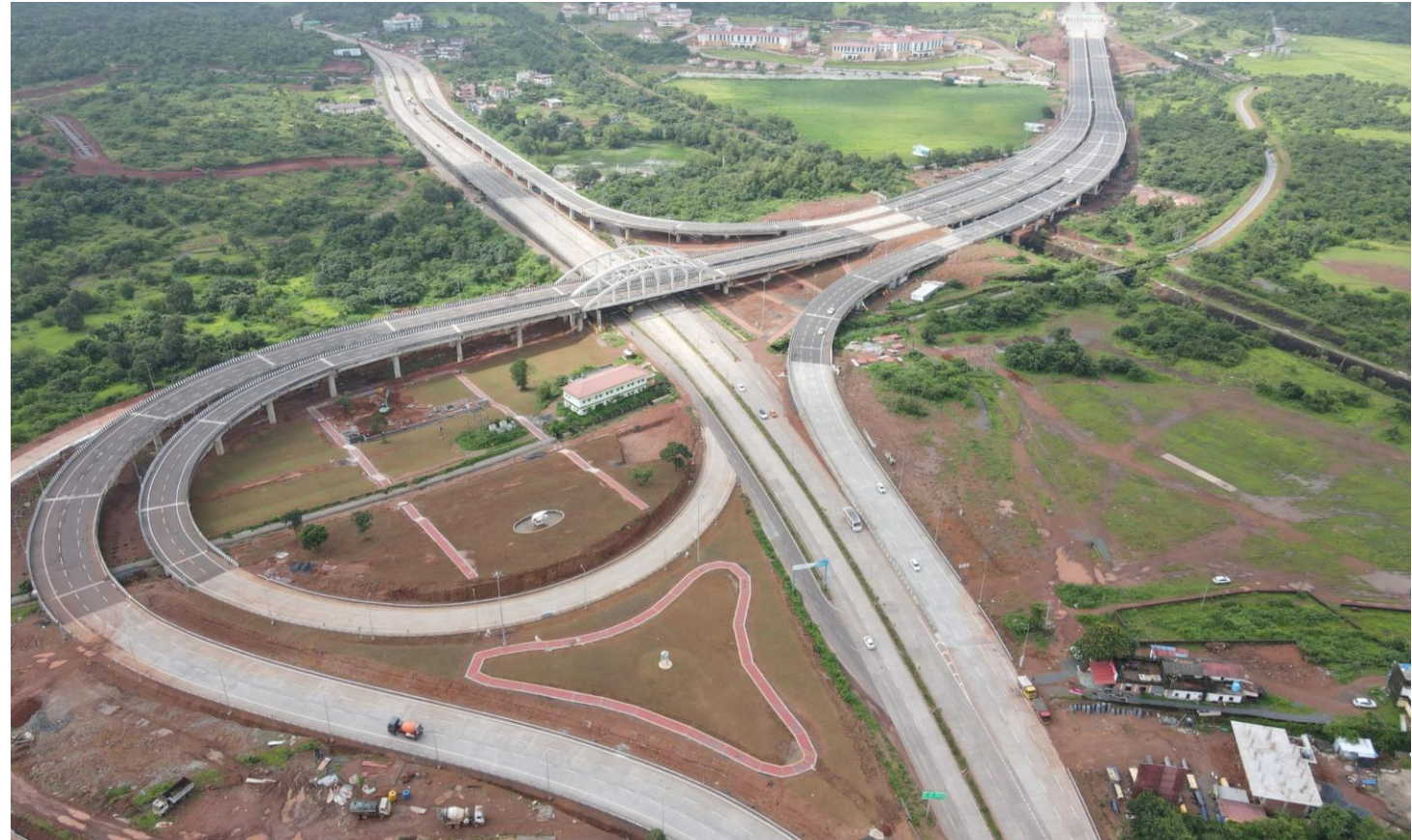
The elevated corridor consists of numerous piers that reach height of up to 40 meters.
